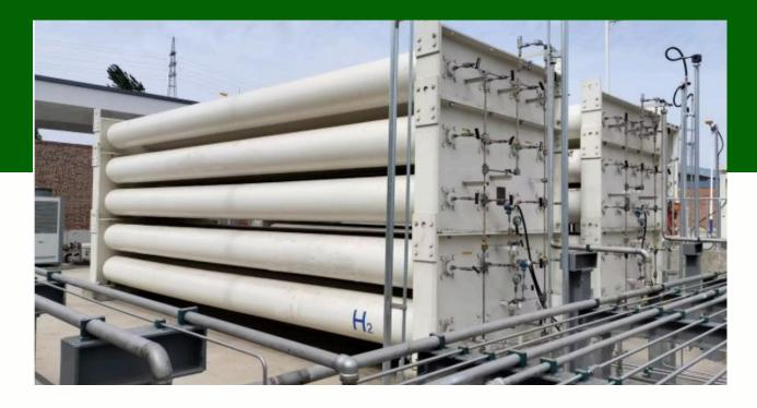
Our hydrogen storage cylinders are designed for high efficiency and safety. With a designed pressure of 50 MPa and operational use at 45 MPa. Depending on the size of the refueling station, the cylinders can be combined to form groups of different total volumes.
